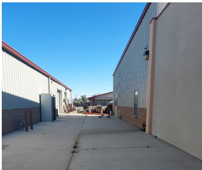
Long uneven alleyway between collections storage, annex, and main museum, which confuses guests and creates issues during inclement weather.
