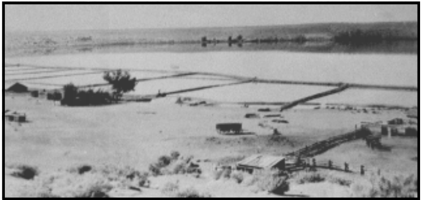
Evaporating ponds at Big Soda Lake can be seen here surrounded by dikes to contain the water.
